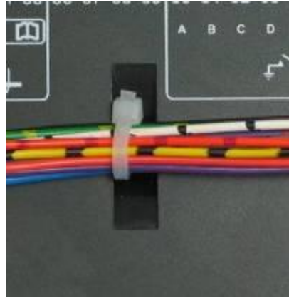
With Cable And Tie In Place
