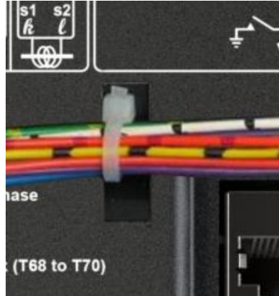
With Cable and Tie in Place
